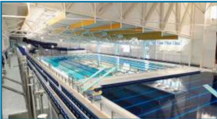
The life centre, Plymouth: Movable floor, vertical bulkhead and disabled platform
