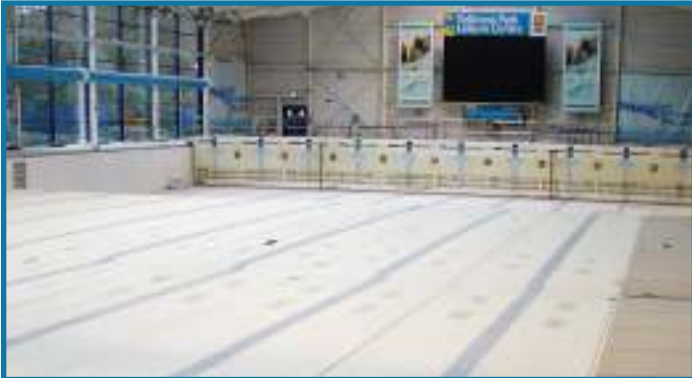
Tollcross Park Leisure Centre, Glasgow: Movable floor and Horizontal bulkhead
