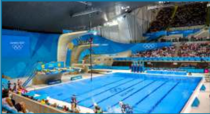
London Aquatic Centre, London: Movable floor, horizontal and vertical bulkhead
