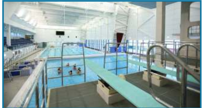
Southend Diving & Leisure Centre: Movable floor
