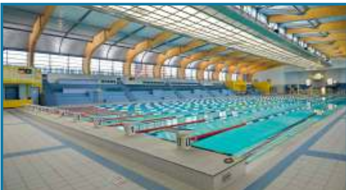
Stadium Park Aquatics, Sunderland: Movable floor and bulkhead
