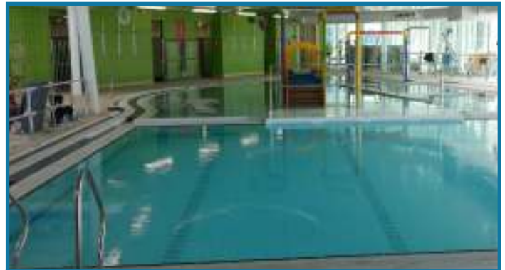
Leisure & Community Heart, Redcar: Movable floor and vertical bulkhead
