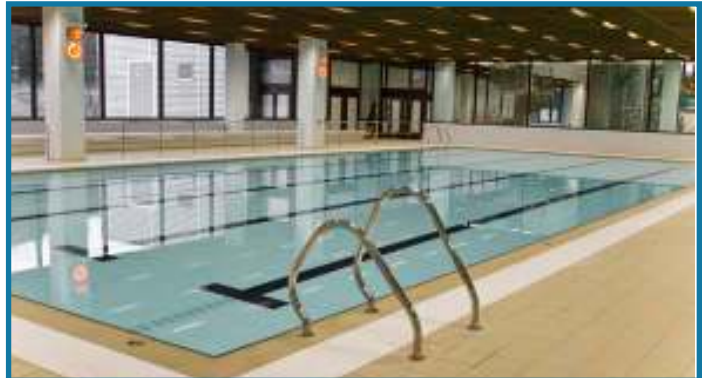
Royal Commonwealth Pools, Edinburgh: Movable floor and bulkhead
